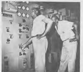
THE RESPONSIBLE job of operating and safeguarding costly turbo-generators lies with M. Dunker, left. Assisting is W. Prime. E TRABAJO responsable di opera y proteha turbo-generator costoso ta keda den man di M. Dunker, robex. Ayudando ta W. Prime.
